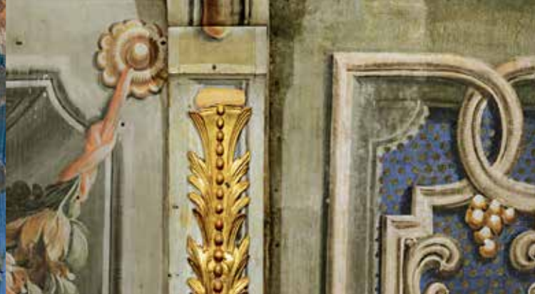
Balustrade of a loge, showing the original colouring following removal of the overpainting
