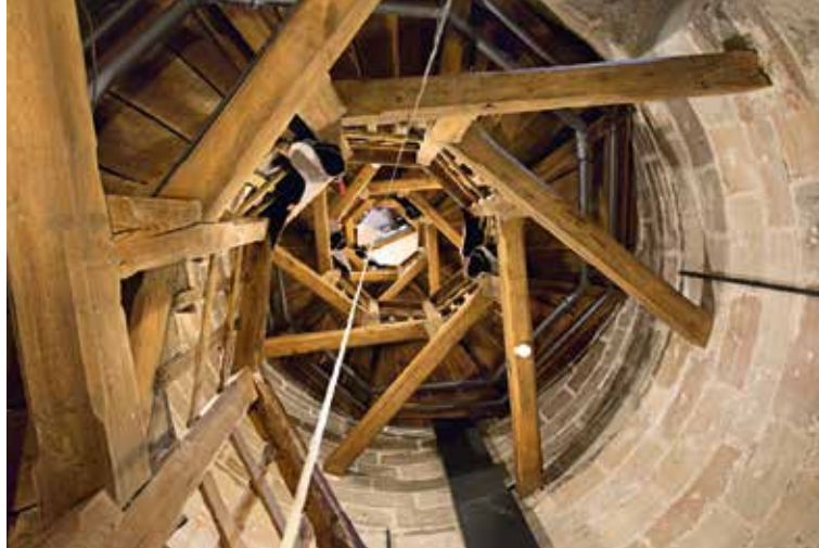
View into the staircase in the Sinwell Tower
